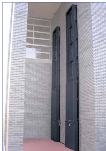
Figure 4. Lift Platform guided in a double column EH/DC.
